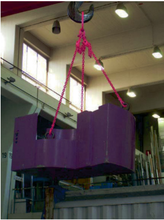
FIG. 3: Lifting an 8 t monochromator shielding part into one of six 20-foot ocean containers inside the service hall of the FRJ-2 reactor.
