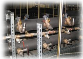
Machine hall raised floor
