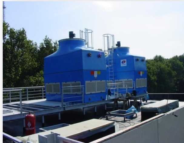
Central cold water supply
