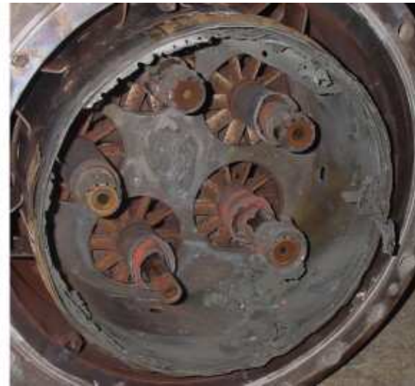
Burner assembly damaged due to combustion instabilities
