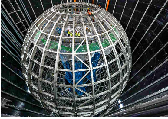
Figure 22: Support structure of the central detector and the installation platform with the workers, photo from June 2022.
