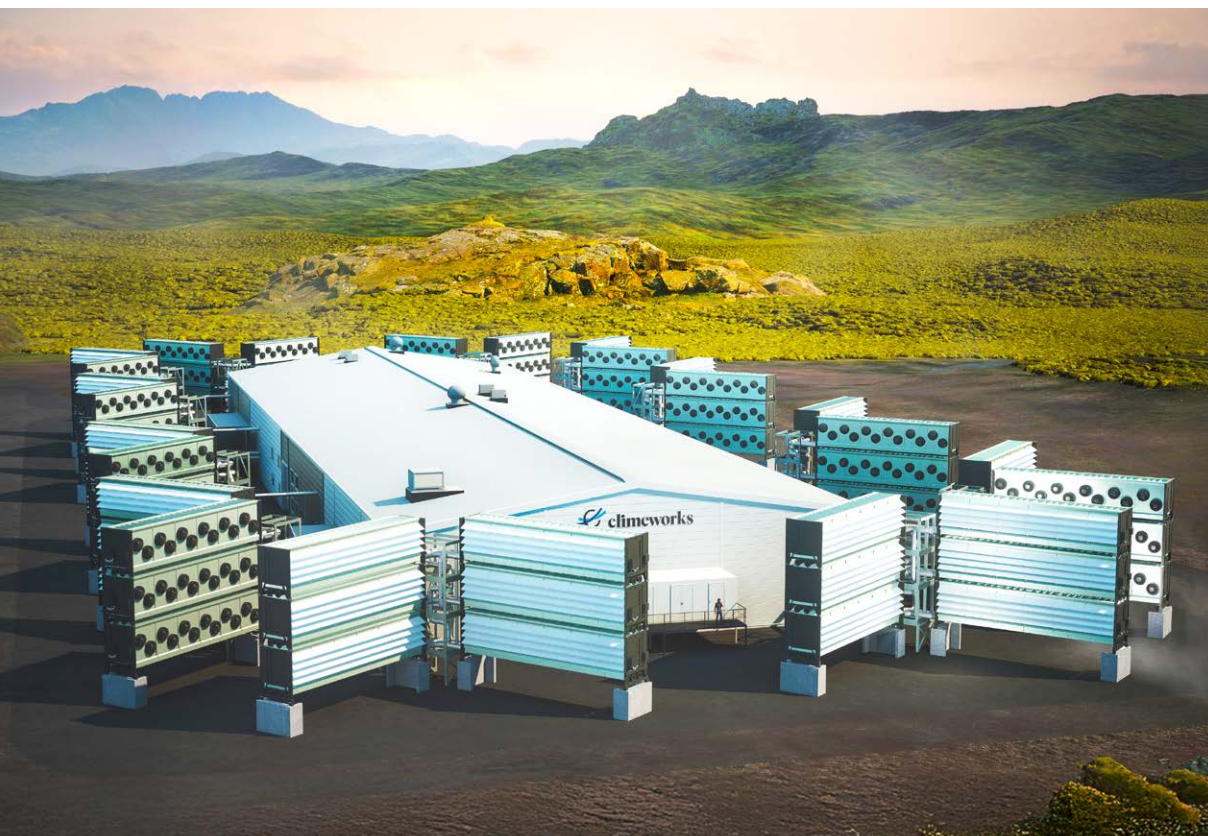
← The collectors, which filter the CO 2 from the air, are housed in large containers in the Mammoth plant. When fully operational, there will be 72 containers.
